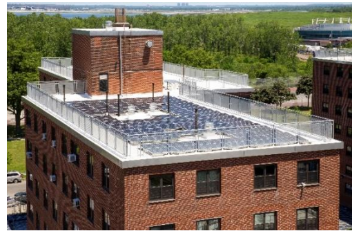
Ocean Bay (Bayside) 修复后的屋顶与太阳能板系统
