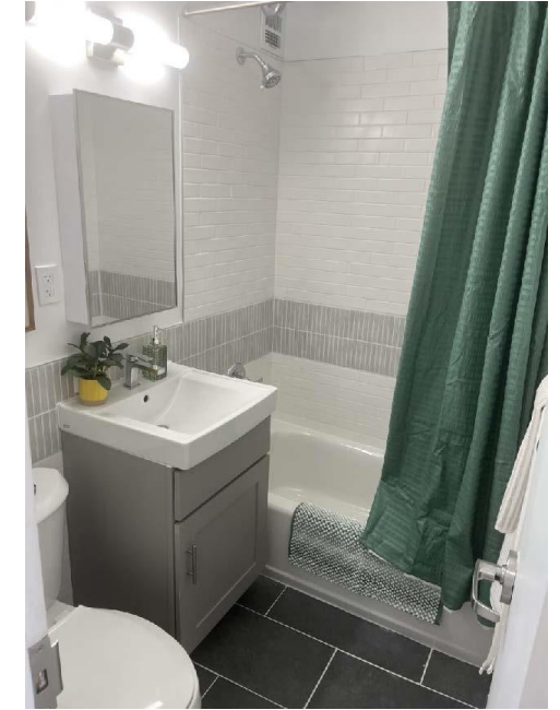
New bathroom fixtures
