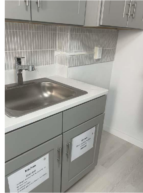
New kitchen cabinets
