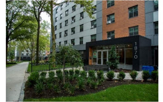
Site improvements at Baychester
